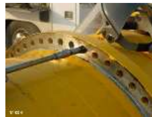
Cleaning paint and rust prior to torquing
