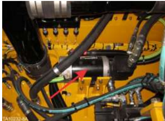
(typical pump(s) located in front, right, inside of rear frame)
